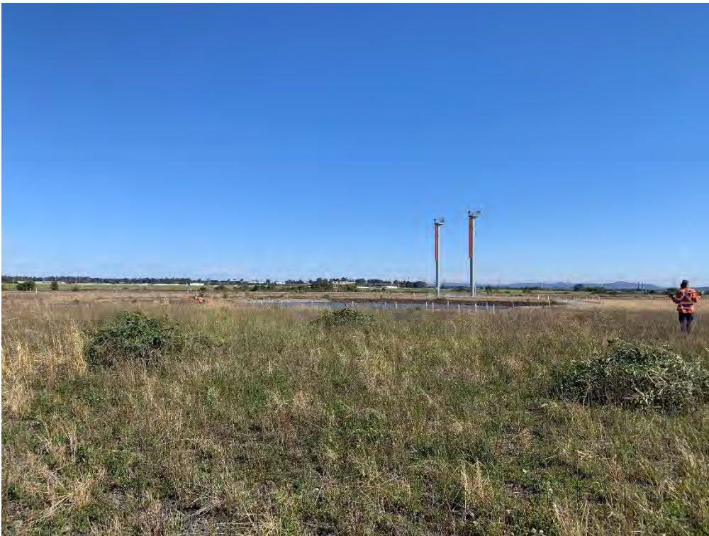
Plate 2: Works area after vegetation removal
