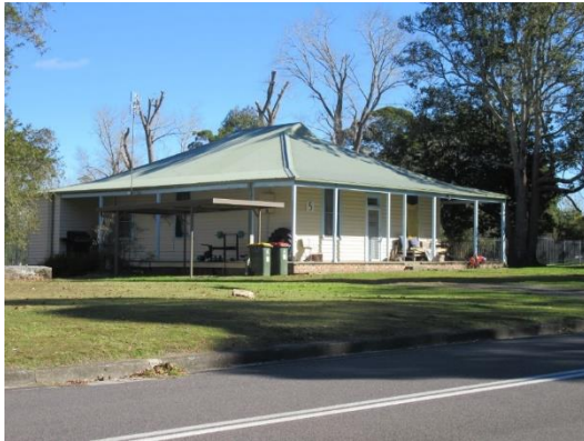
Building 5 – staff accommodation, 1912-1913
