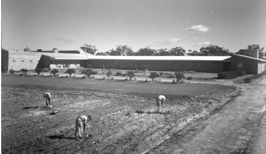
19 The sub-institution (Building 10) after conversion to the Privilege Cottage, 1948. Source: SLNSW d1_43228h.
