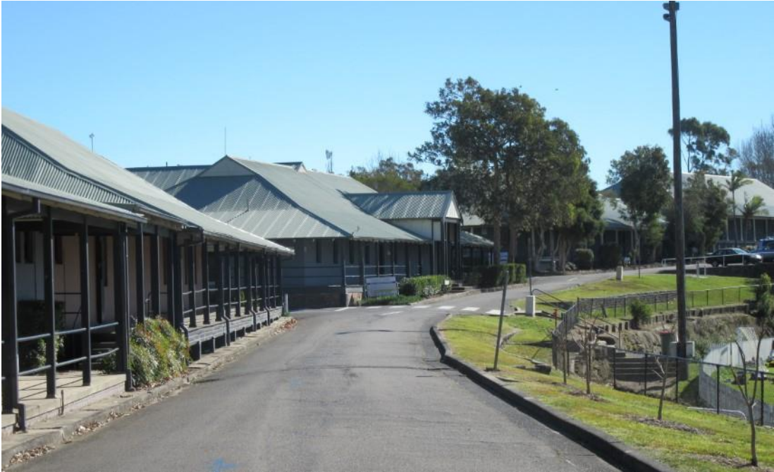
26 Looking north along The Avenue. Early administration and dormitory buildings form a memorable composition as the road curves and rises above the cricket oval to its east.
