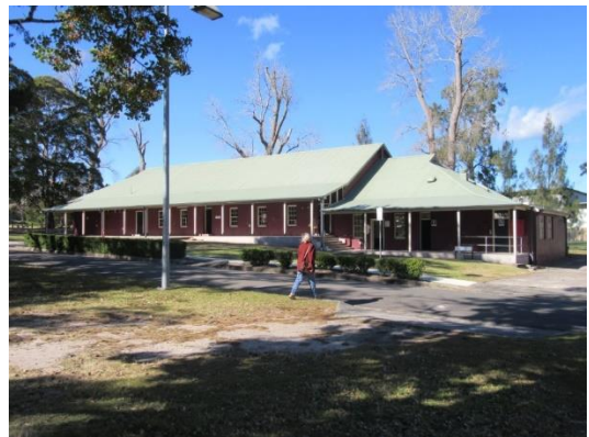
Building 21 – dormitory, circa 1913
