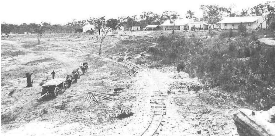
9 One of the tramlines linking the quarries to building sites. Temporary buildings can be seen in the background.
