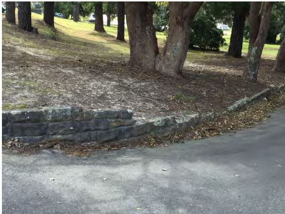
Figure 9: Stone retaining wall adjacent to The Avenue
