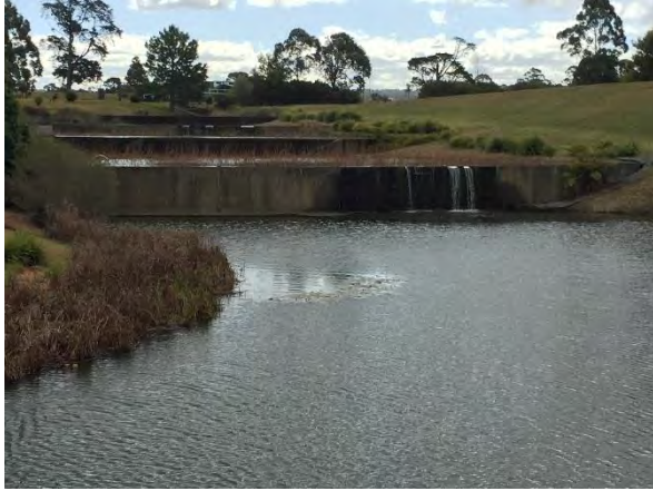
Figure 13: Tiered dam in the Parklands, view north
