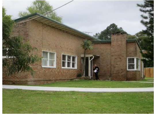
Building 8 - staff cottage attached to sub-institution/Privilege Cottage, 1944
