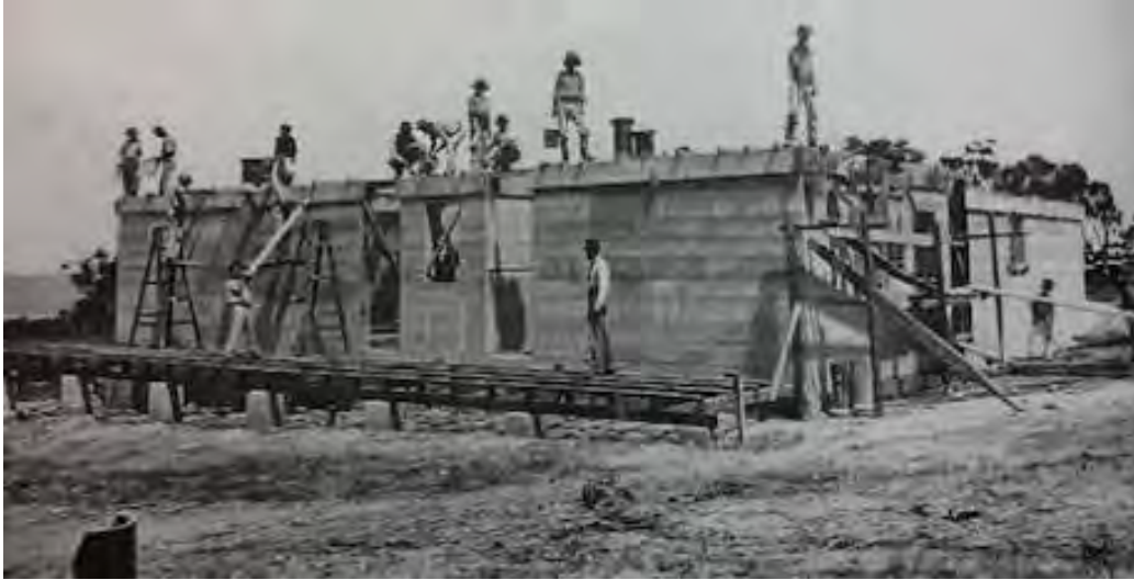
Figure 9: Construction of the residence for the Superintendent, 1912 (Image DCS/DJJ HC)
