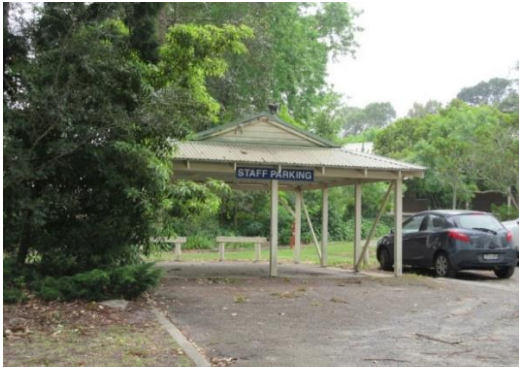
Carport to the south-east of Building 19
