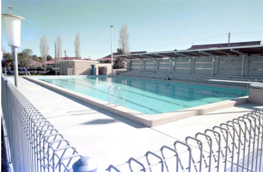
22 The newly completed swimming pool (Building 47), July 1973. Source: SLNSW d3_48546h.
