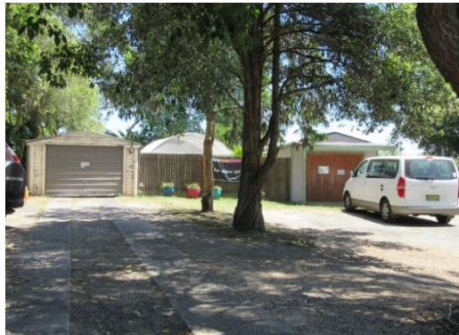
Garages to the north of Building 2
