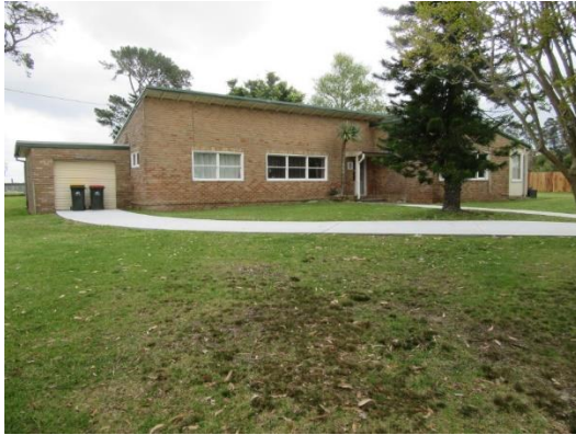
Building 7 – staff cottage attached to sub-institution/Privilege Cottage, 1944
