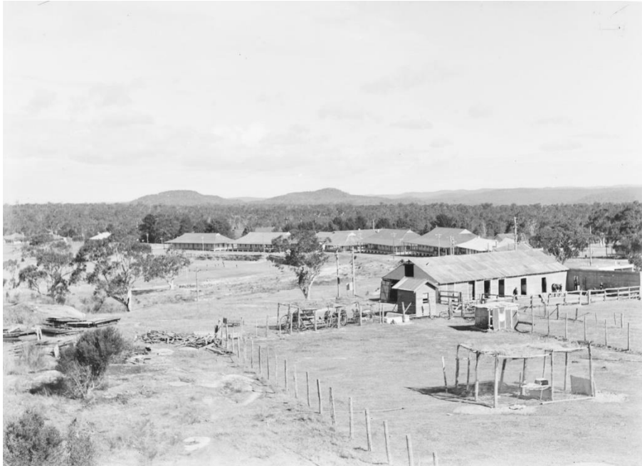
15 Looking south towards the range of dormitories along what is now known as The Avenue. The original dairy is in the foreground. The photograph was taken in July 1938.
