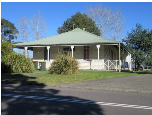
Building 3 – staff accommodation, 1912-1913
