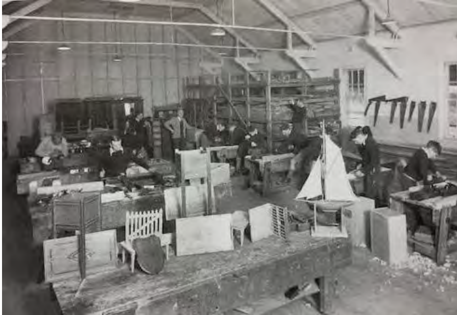
Figure 15: Carpentry workshop, 1938 (Image State Library of NSW)
