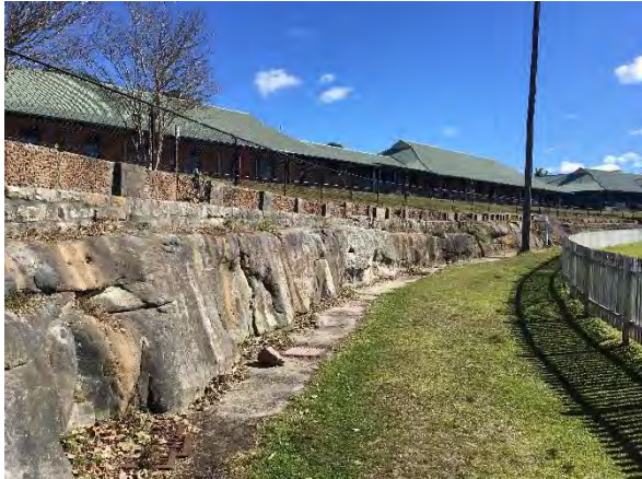
Figure 7: Cutting adjacent to the oval with dormitories behind
