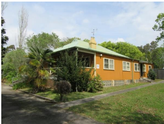
Building 9 - Assistant Superintendent's Residence/ Superintendent's Residence, 1912
