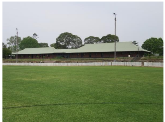
Building 25 and 26 – dormitories, 1912
