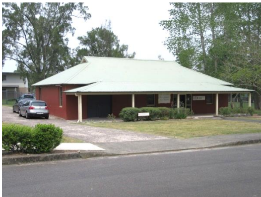
Building 22 – maintenance store, 1912-1915
