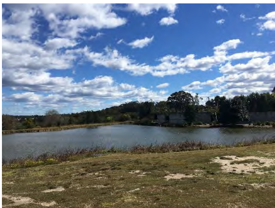
Figure 8: Large dam associated with the nearby Mt Penang Gardens, facing northwest
