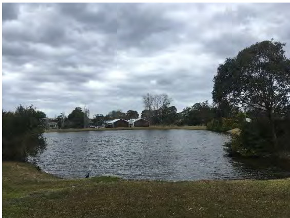
Figure 14: The dam located in the central portion of the study area, facing north
