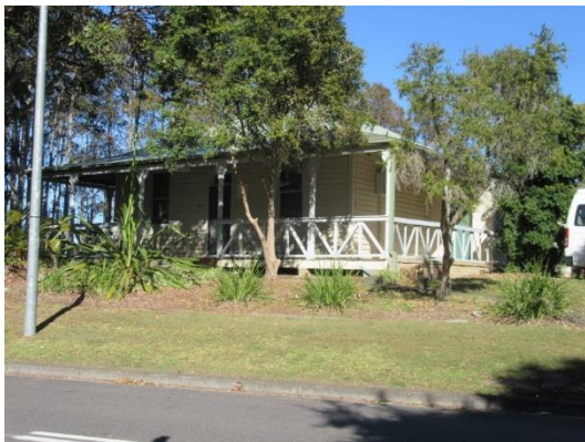
Building 1 - staff accommodation, 1912-1913
