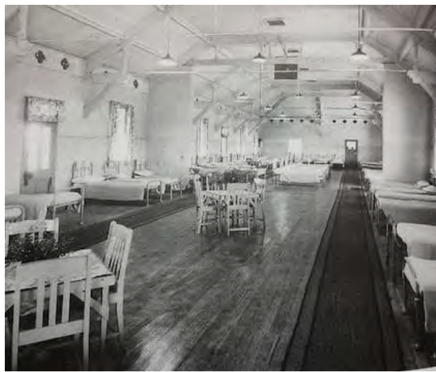
Figure 17: Dormitory following refurbishment, 1948 (Image State Library of NSW)
