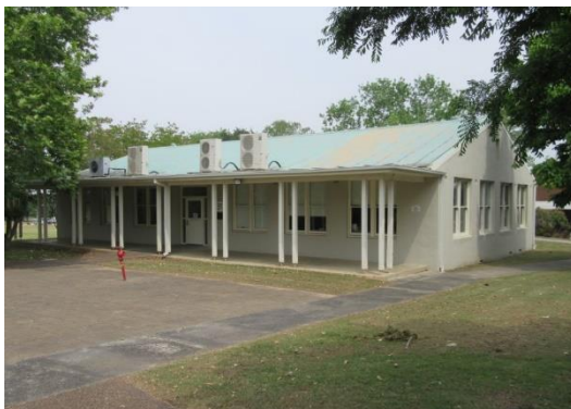
Building 31 – dining room and main kitchen, circa 1950
