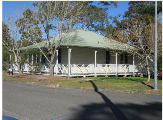
Building 6 – staff accommodation, 1912-1913
