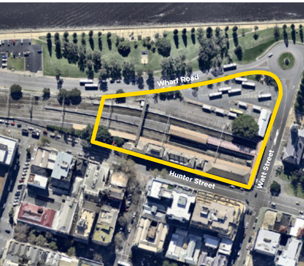
Newcastle Station precinct
